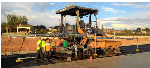
Figure 1: The Big Sonic-Ski from Moba with four CAN-connected sensors for asphalt paving (Source: Moba)
