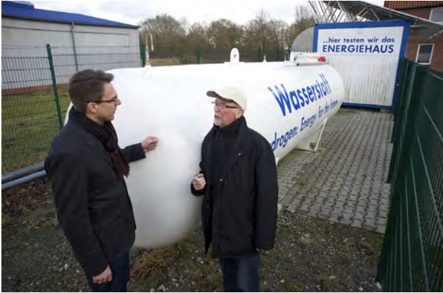
Figure 3: Fuel from the hydrogen tank: The Blue Hamster can completely supply a company, whose electrical consumption is less than 100 000 kW hours per year, with clean, solar energy; that which is squirreled away in the summer can be used during the winter (Photo: Thomas Fröhling/vor-ort-foto.de)
