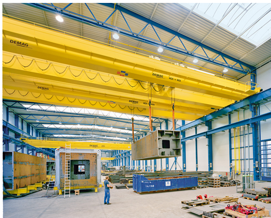
Figure 1: Electric Overhead Traveling cranes (Photo DEMAG)
