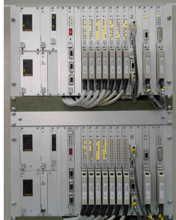
Figure 3: Vehicle control unit (VCU)
