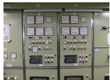
Fig. 1: Monitoring and control of automation subsystems in large scale systems may comprise 20.000 of I/O-points. Photo: Kongsberg Norcontrol (first; Berge Nord, second & third; Main switchboard outside & inside)
